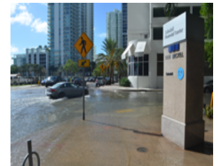
Figure 2: Sunny day flooding, Miami October 2016
